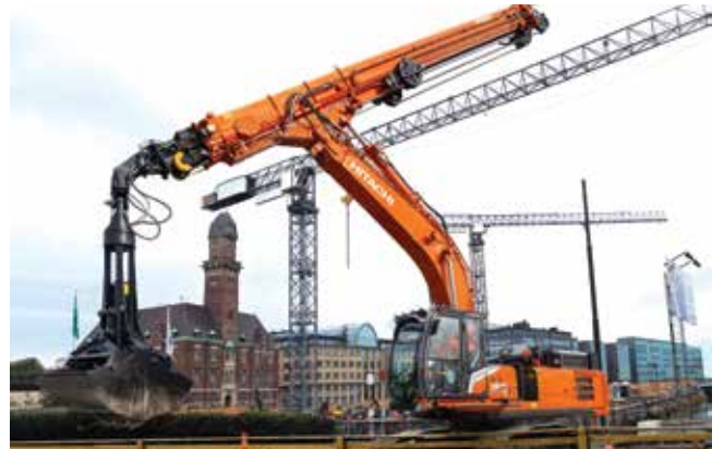
Special application excavators
